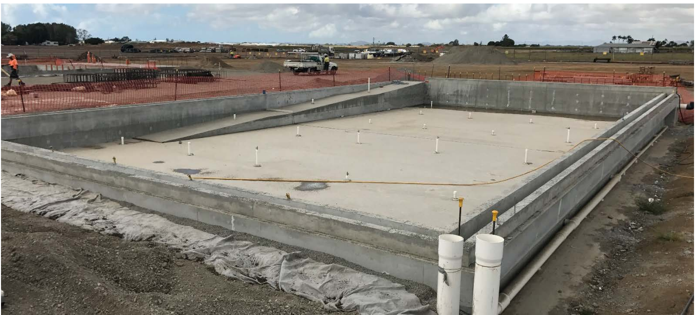
Figure 2 - 25m pool shell
