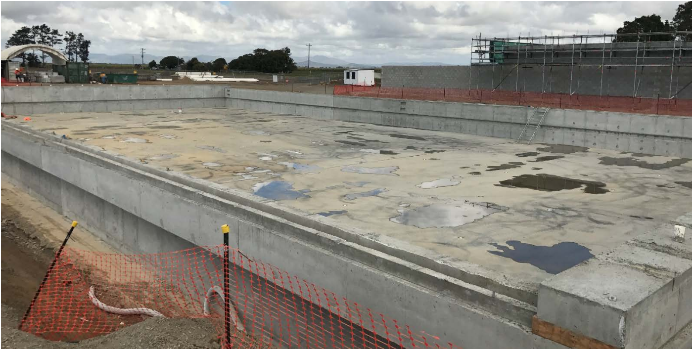
Figure 1 - 50m pool shell with pool plant building in background
